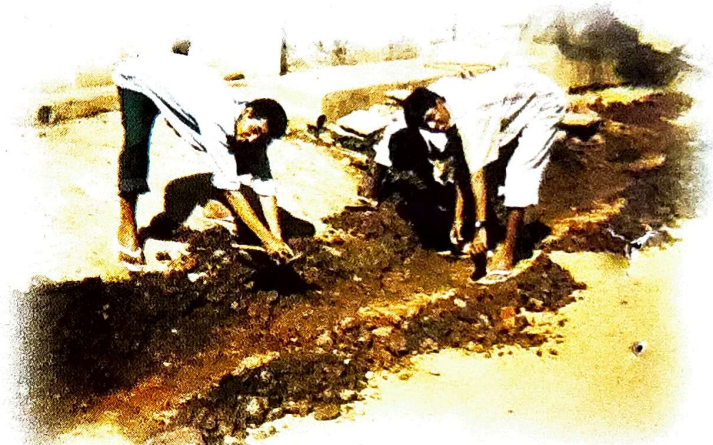
NSS: Drainage Construction Work at Kandrika
